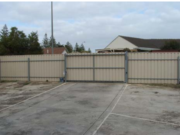
View of rear security gate - access to car parks.
