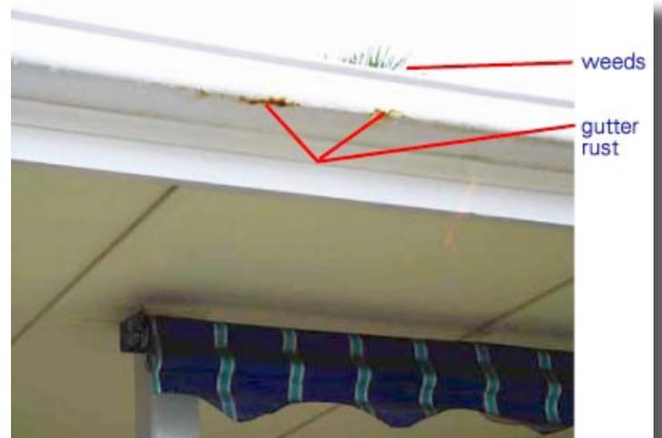
photo we see weeds in the gutter. This has led to rusting from the inside of the gutter. This is the result of many years of neglect. This gutter section will need replacing.
