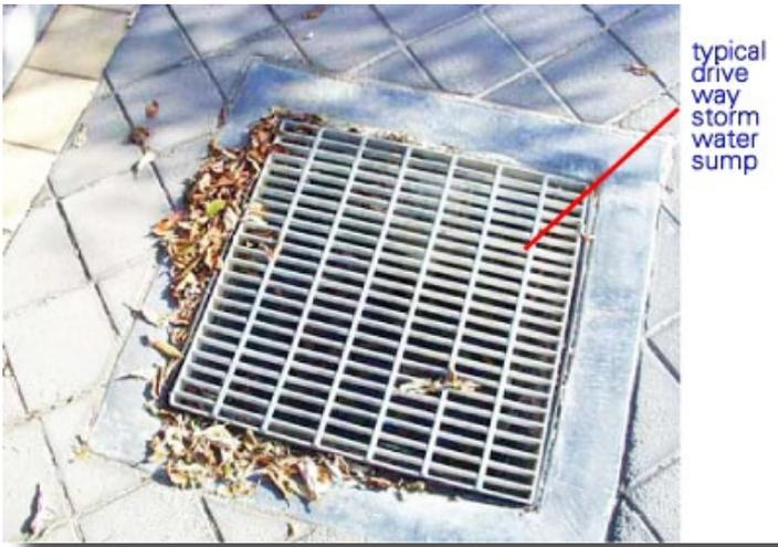
In the above photo is an example of a stormwater sump. These are commonly found in driveways. They take surface water down to the drainage pipes at the bottom of the sump. These pipes come from downpipes and other sumps. They eventually drain to the street. Over time these sumps fill up with leaves and rubbish. They need to be cleaned out when the gutters are cleaned and as needed.
