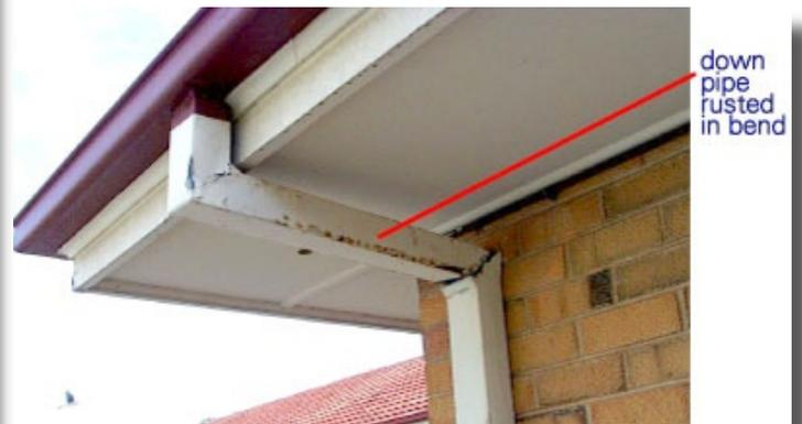
In the above photo we see rust in the downpipe serving the gutter above. This is caused by leaf and other waste laying in the pipe over years.
